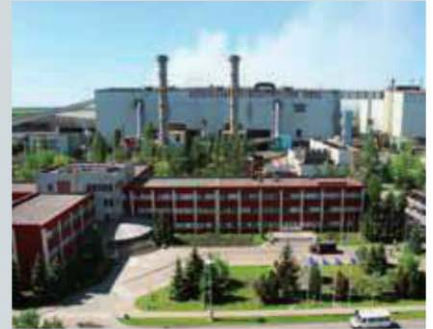
State-owned BMZ was founded in 1984. The current project with Siemens is part of a modernization program that will be running until 2015
