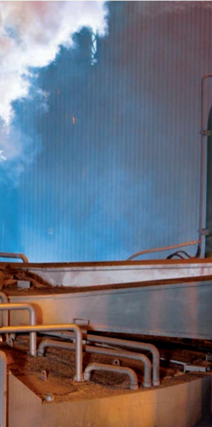
Fig. 1: High-performance electric steelmaking with the most advanced electrode control system
